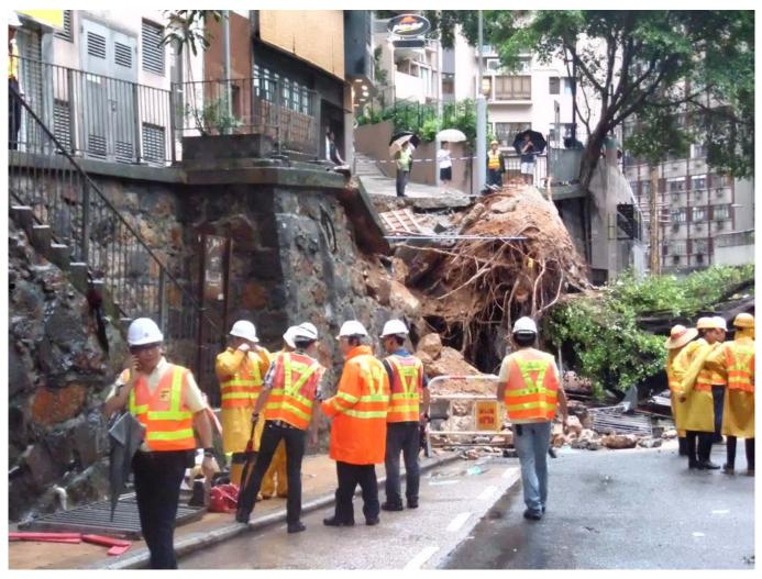
Photo 2.2 – Stonewall Damaged together with Tree T2
